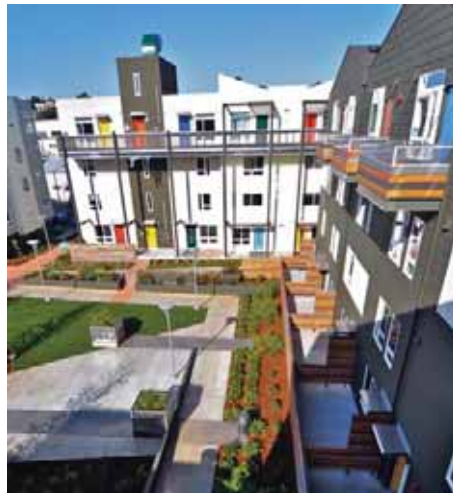
Courtyard Building Illustrative Photo
