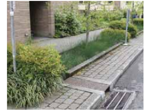
Parkway with Infiltration
