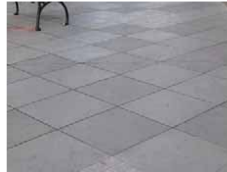
Poured, Scored Concrete
