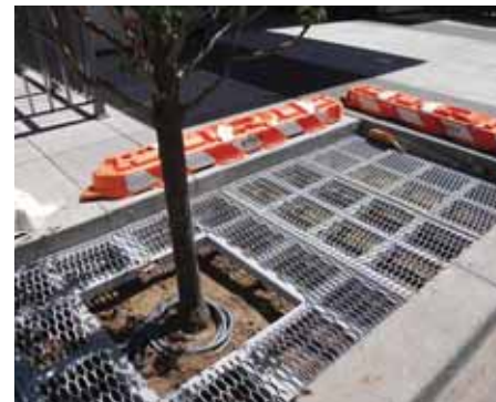
Inground Planter Under Construction
