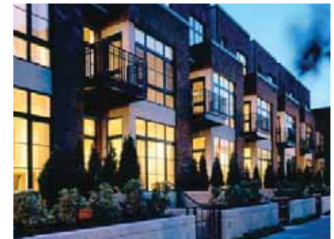
Encroaching Habitable Space (4.5.9)
