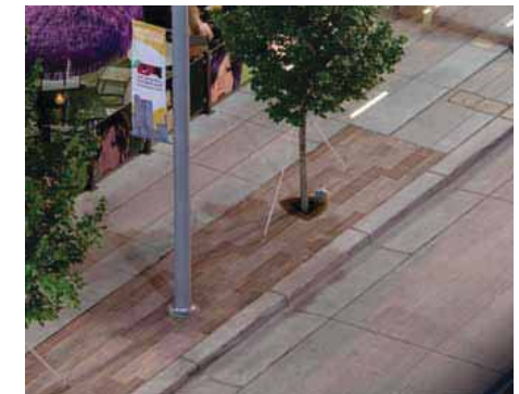
Inground Planter with Paving Installed
