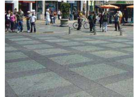
Decorative Concrete Crosswalk
