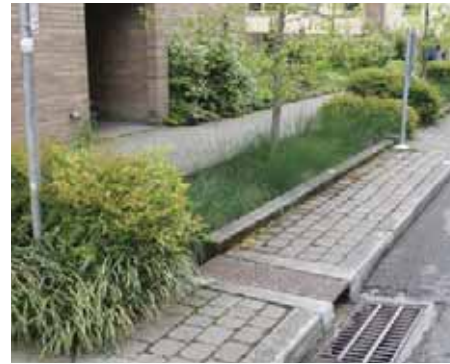
Parkway with Infiltration
