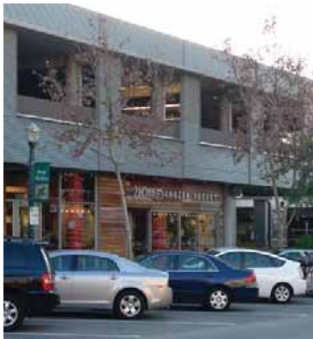
Exposed Garage Building Illustrative Photo
