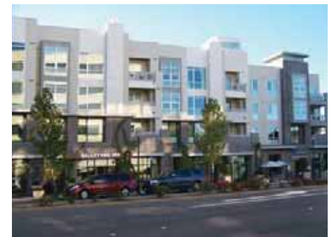
Facade Plane Breaks (4.5.1)
